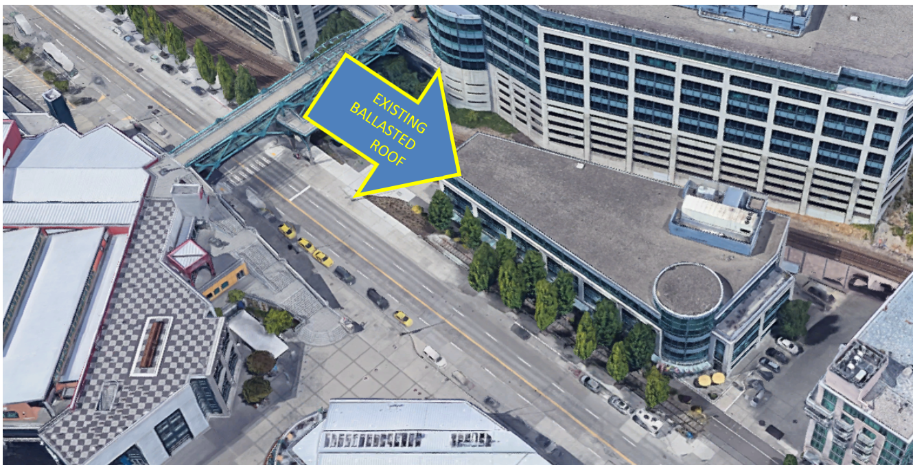
Figure 1. WTCW Roof Replacement Project
